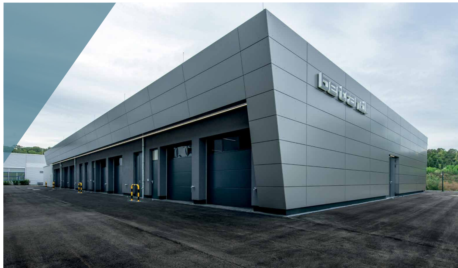
The Bertrandt high-voltage test centre can be used by all our customers.
